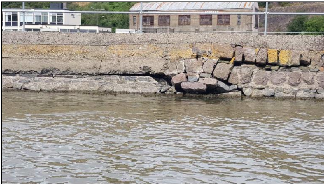
Plate 2.7 Defects on the existing quay wall – Dislodgement of blocks, mortar washout, several phases of wall upgrades (Ch. 550)
