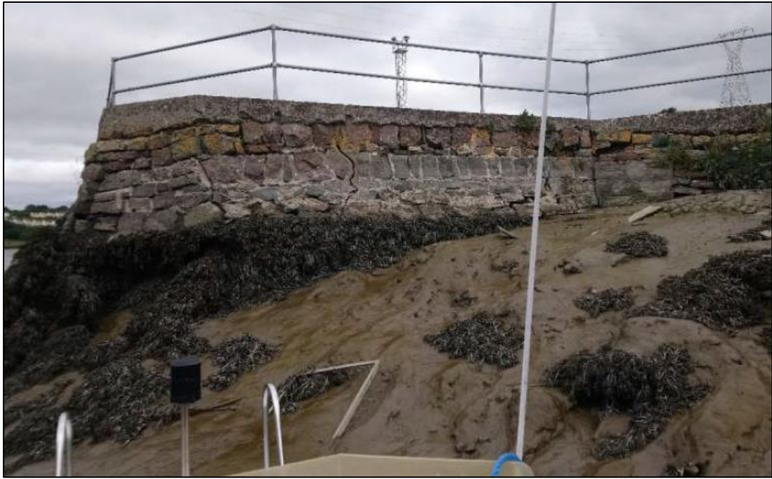
Plate 2.6 Defects on the existing quay wall – large displacement and rotation of the wall (Ch. 540)
