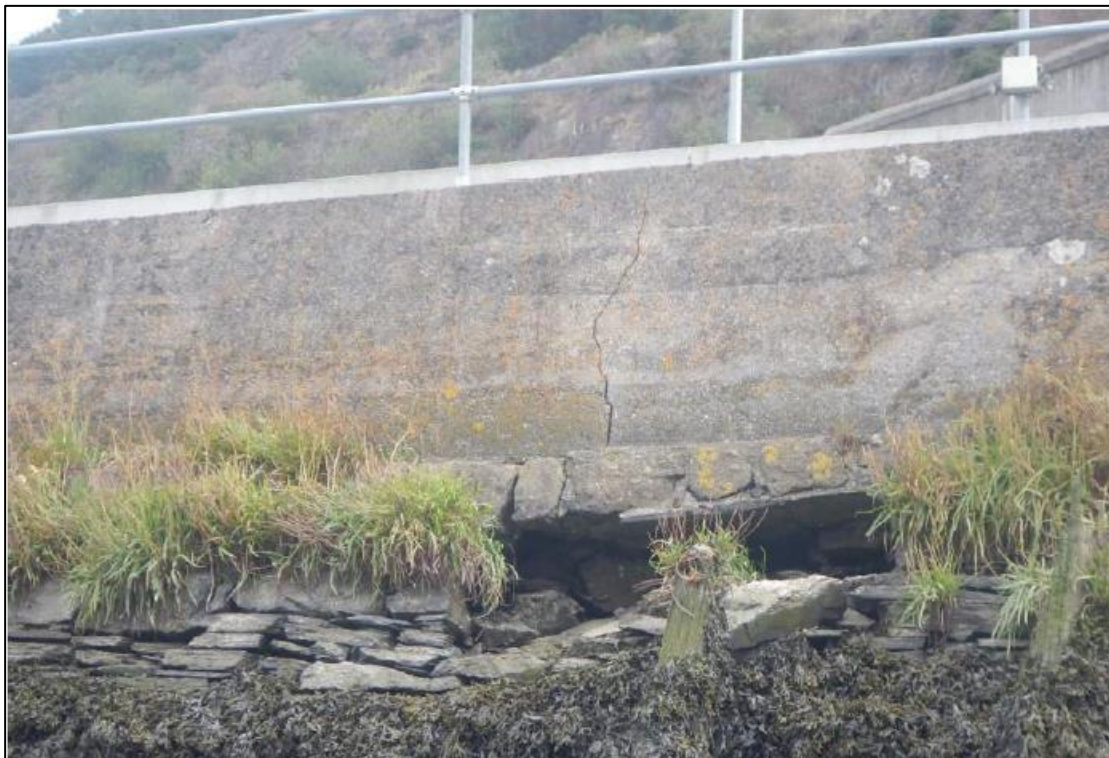
Plate 2.5 Defects on the existing quay wall – cracking of the wall and dislodgement of masonry blocks (Ch. 370)
